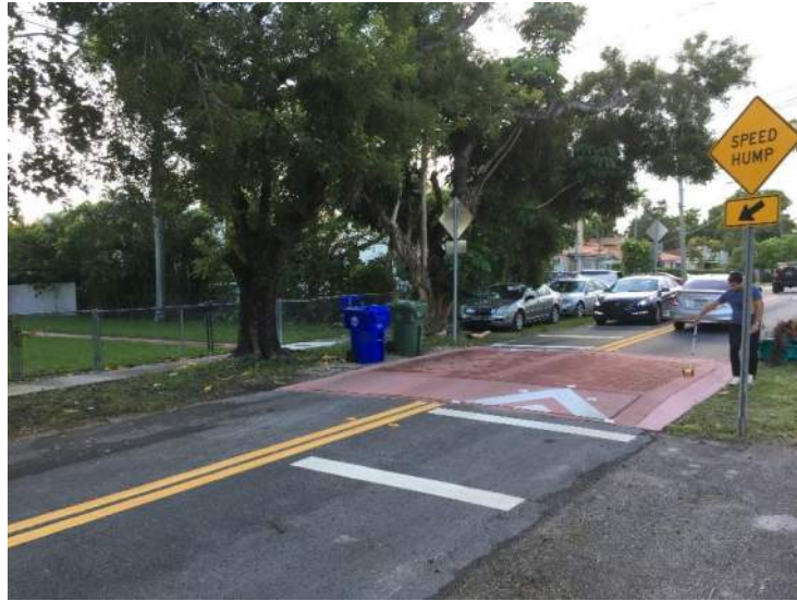
Existing Speed Table (SW 20 th Street)
