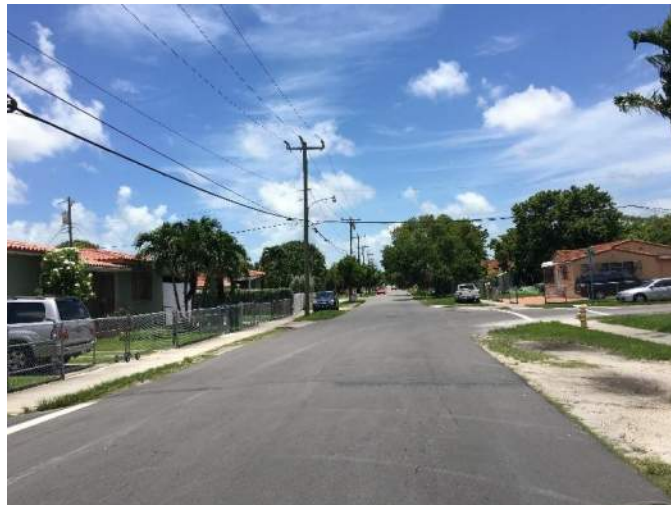
Typical Neighborhood Street (Southbound SW 24 th Avenue north of SW 11 th Street)
