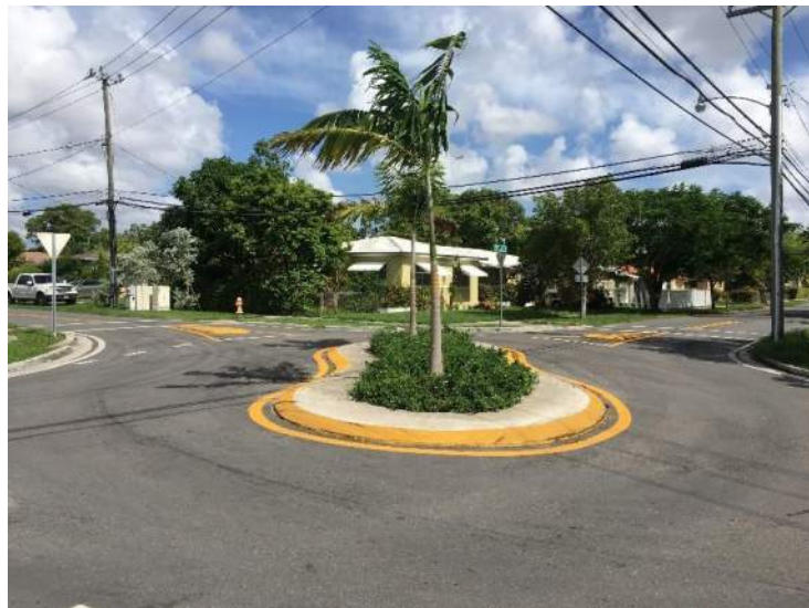
Existing Roundabout (SW 18 th Street and SW 24 th Avenue)
